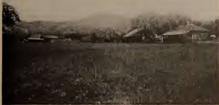
GENERAL VIEW OF FORT MILLER
